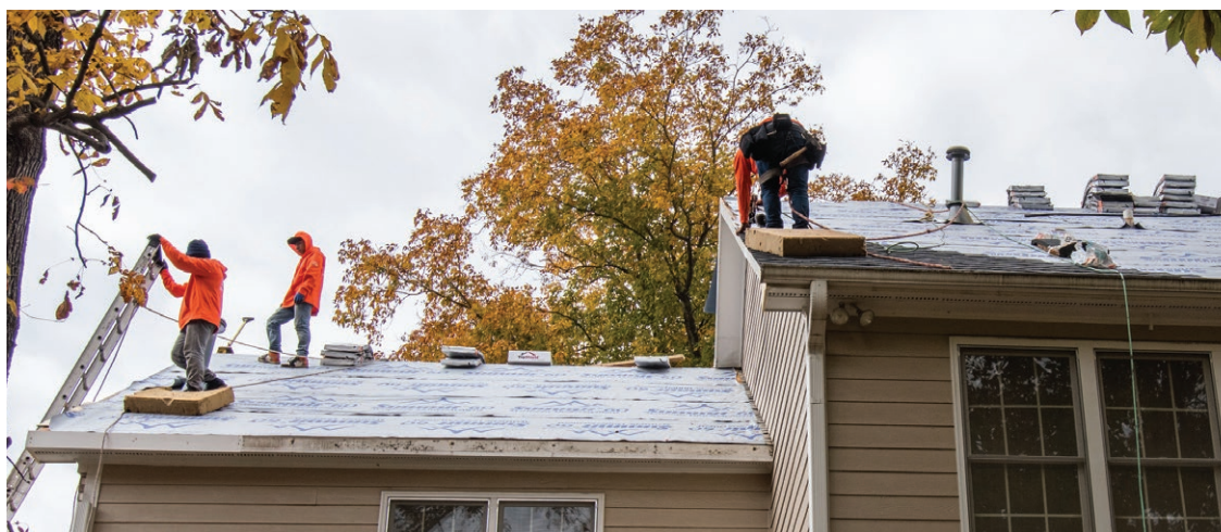
Roofing Renovations depends solely on referrals and networking to build its business.
